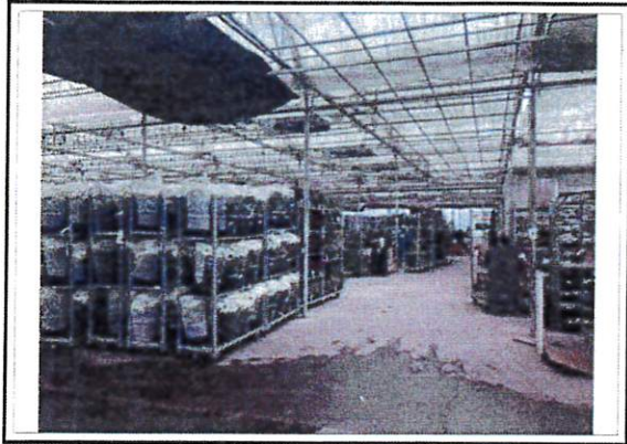
View of Production House
