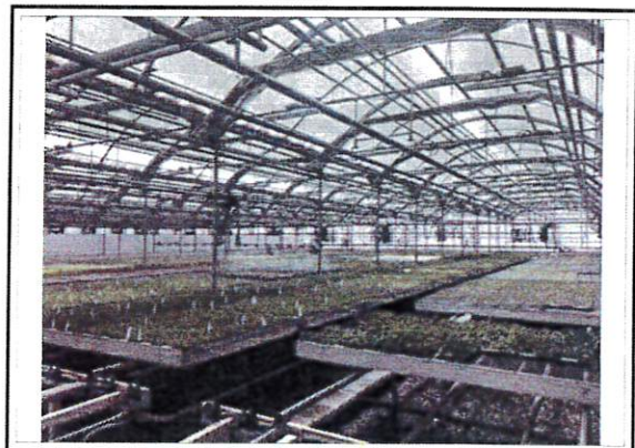
View of Table House
