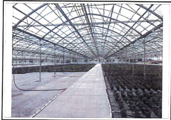
View of S-1 Interior
