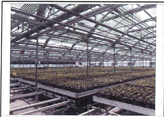
View of Table House
