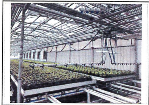
View of Table House
