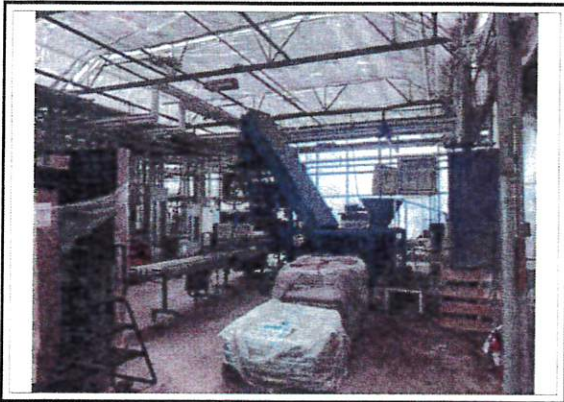
View of Production House
