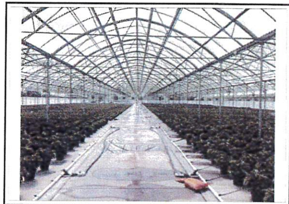
View of S-3 Interior
