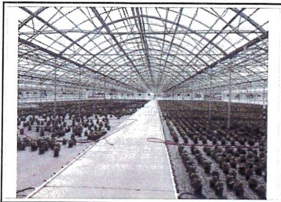
View of S-2 Interior
