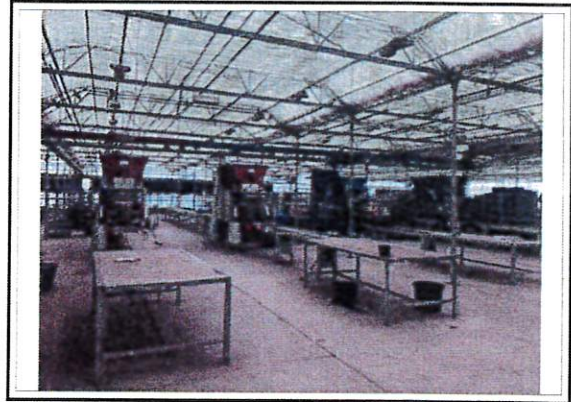
View of Production House
